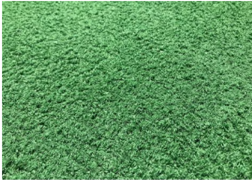
Carpet wear & poor repairs
